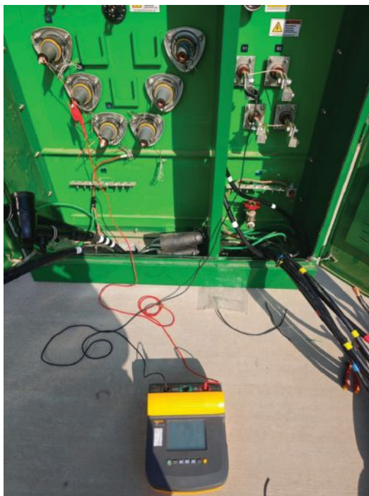
Figure 1: Transformer Insulation Resistance (IR) Testing Connections
