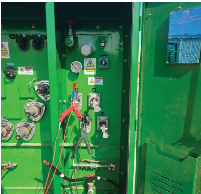
Figure 2: Transformer Winding Resistance (WR) Testing Connections
