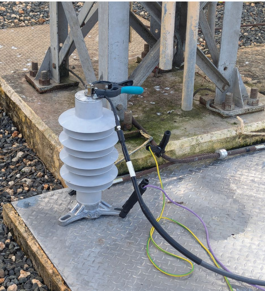
New Surge Arrester Under Test
