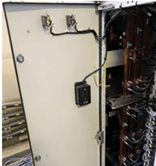
Figure 2: A compact camera is attached magnetically to a panel door, with Ethernet providing communication and power.
