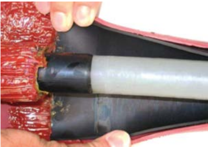
Figure 3: PD inside a Cable Termination
