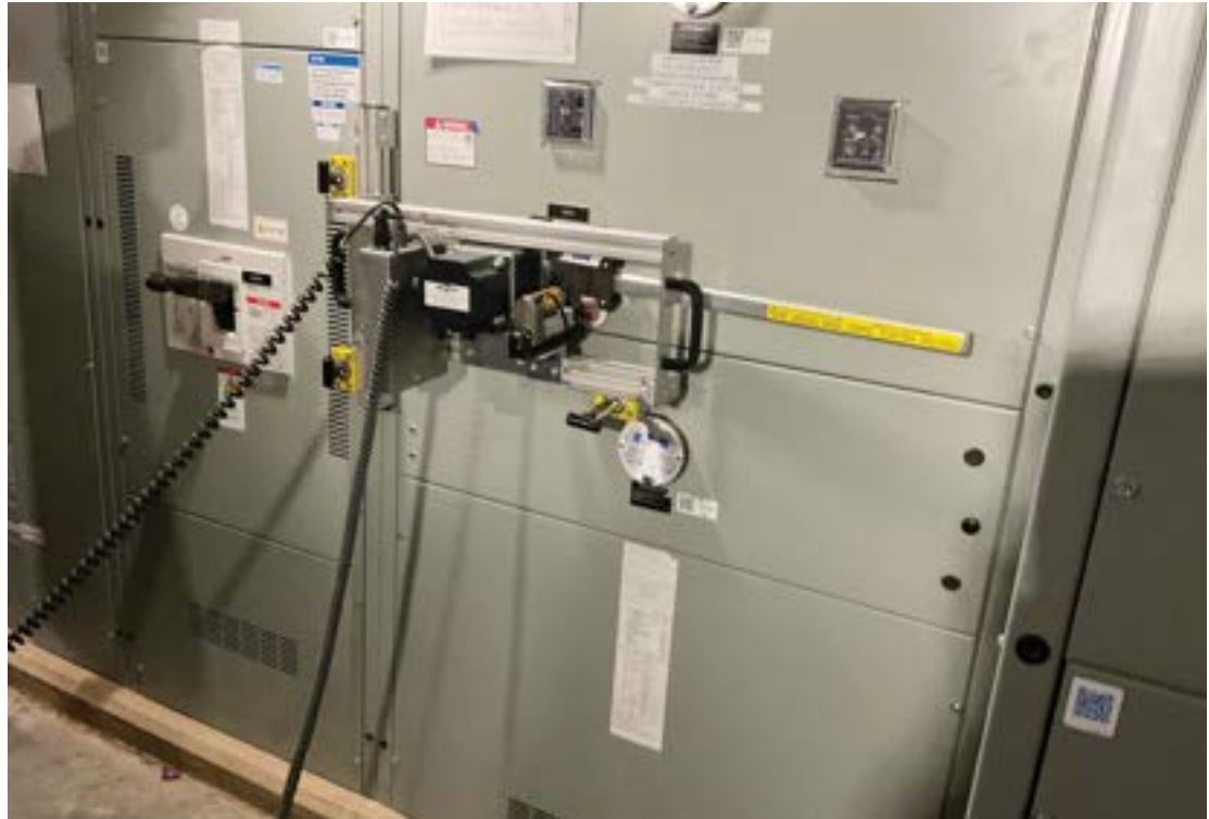
Figure 5: Bolted Pressure Switch Operator RSA-135 by ArcSafe
