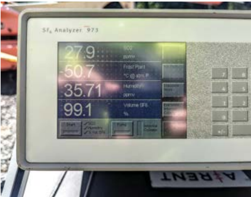
Figure 7: Results of SF 6 Gas Analysis Showing Elevated Sulfur Dioxide
