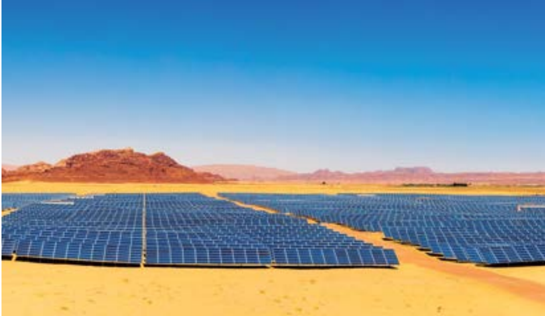
Quweira Solar Power Plant, Jordan
