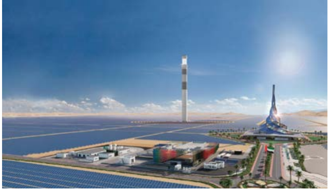
Mohammed bin Rashid Al Maktoum Solar Park, UAE
