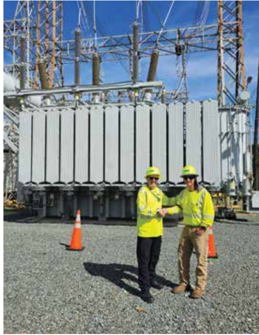
Completion of Commissioning of Power Transformer in Puerto Rico
