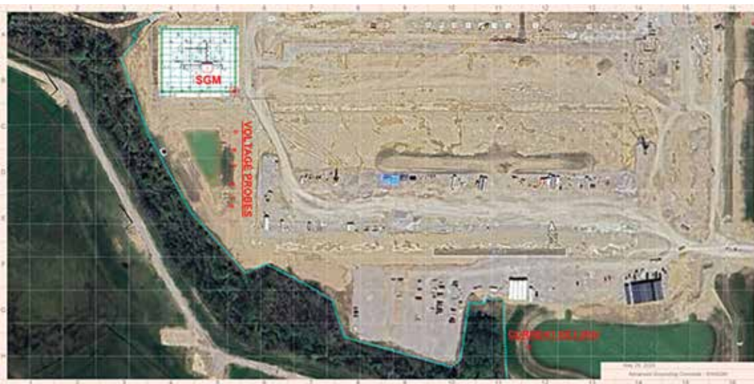
Figure 1: Data Center Substation, Ohio, Using Computer-Based Multimeter
