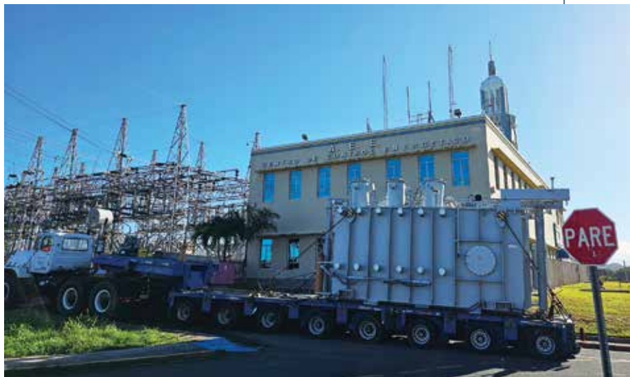
Substation Construction in Puerto Rico
