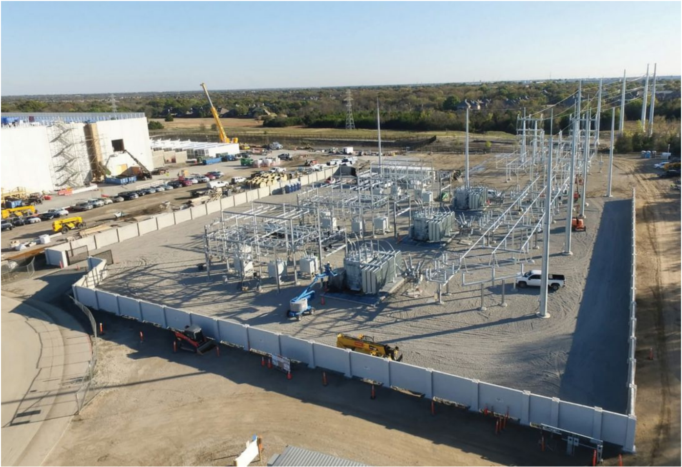
Photo 8: Commissioning a Service Entrance in a 138-kV Substation
