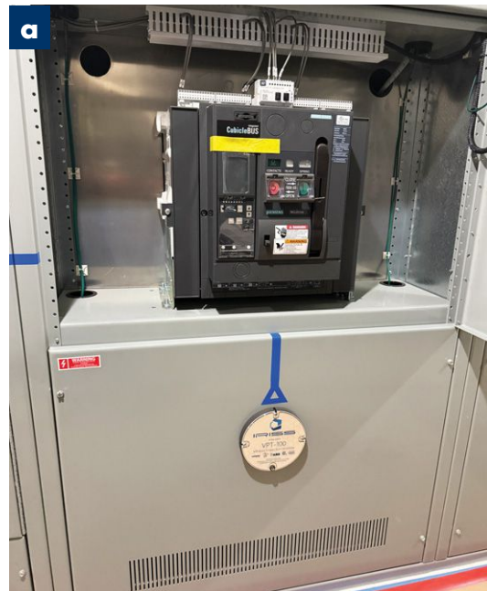
Photo 2: This bolt-in LVCB (a) cannot be removed due to the (b) enclosure wall.
