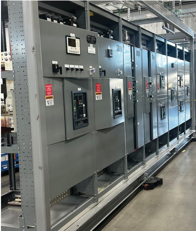
Photo 1: A Modular Skid Assembled in the Factory
