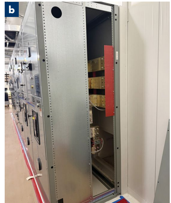
Photo 2: This bolt-in LVCB (a) cannot be removed due to the (b) enclosure wall.
