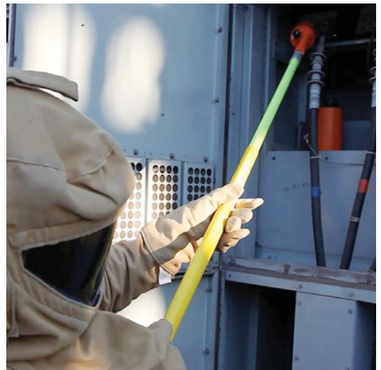
Figure 4: Medium-Voltage Non-Contact Probe
